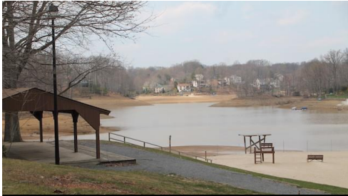
Figure 4-4d. Emergency Spillway Project
