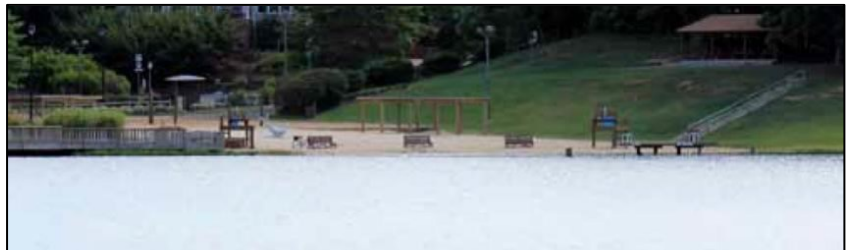
Figure 4.6. Lake Montclair emergency spillway dual-use as Dolphin Beach prior to 2018 modification to increase storm water surge capacity.
